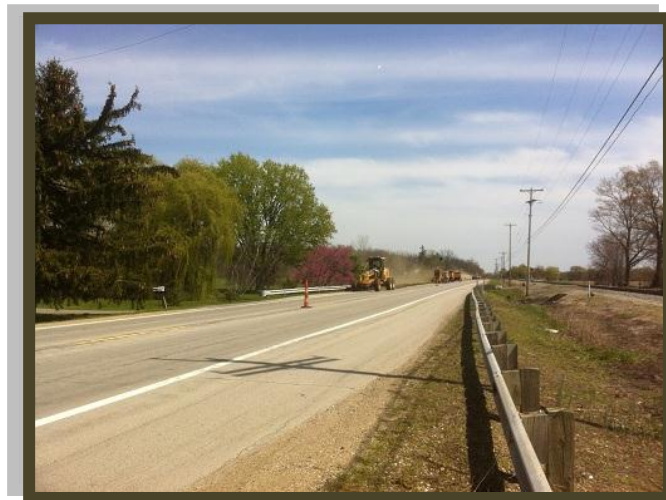
Shoulder Maintenance Operation
